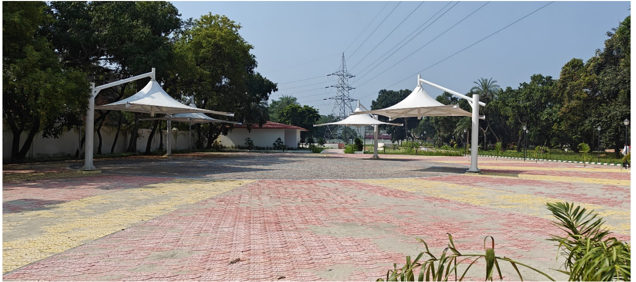
Central lounge area, with four all-weather tensile automatic roofing structures
